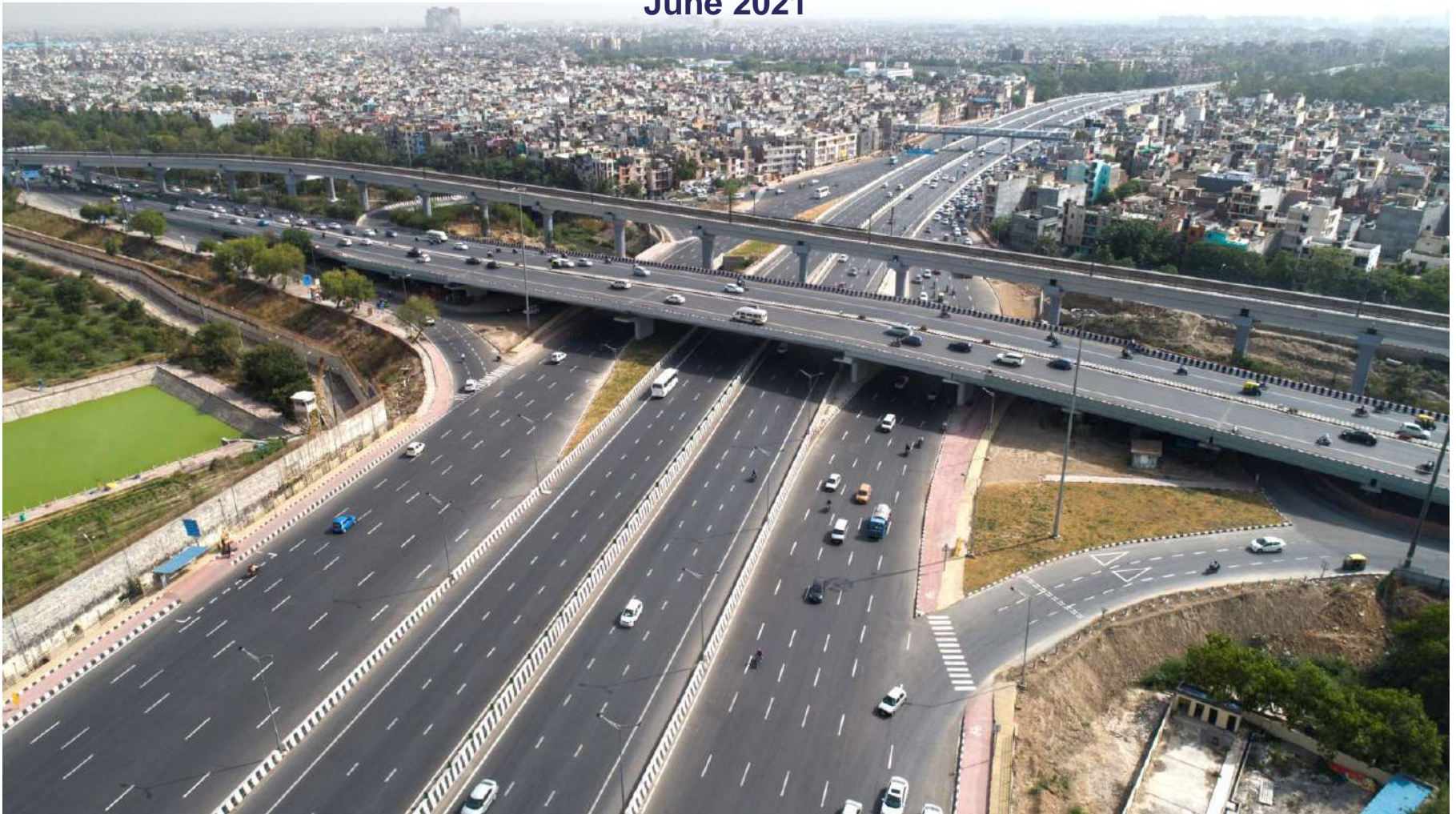
Actual photo of Delhi-Meerut Expressway; completed in record 19 months vs. scheduled 30 months
